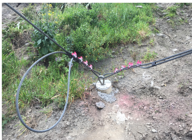
Figure 6.42. An example of a localised concrete head detail to support the upslope anchorage (NCTIR, 2019)
