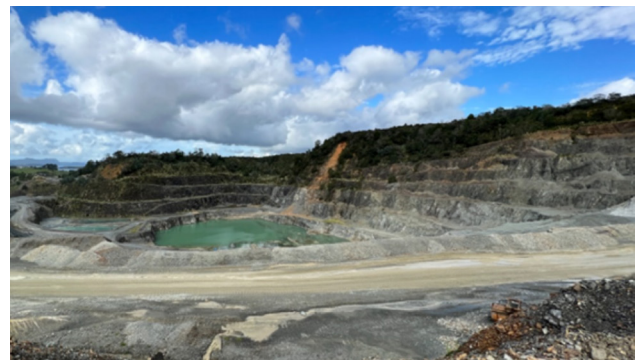
Figure 6.20. Bench and batter rock slope profile in Otaika Quarry (Source: Winstone Quarries)
