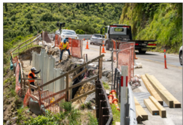
Figure 6.8. SH23, Remutaka Hill Underslip Repair (Source: NZTA Waka Kotahi, November 2024)
