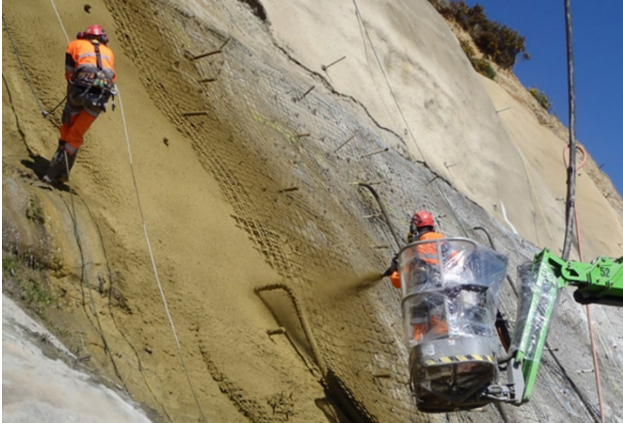
Figure 6.25. Sprayed concrete combined with steel mesh at Rock Road, Nelson (Source: Ground Anchor Systems)
