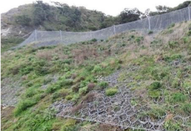
Figure 6.48. An example of the impact vegetation growth can have when developing within the dynamic section of the structure (NZ Transport Agency Rockfall Protection Design Guideline, 2023)
