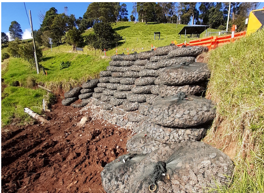
Figure 8.2. Rock bags used to reduce risk of further land movement and undermining of road (Bluemont, 2025)
