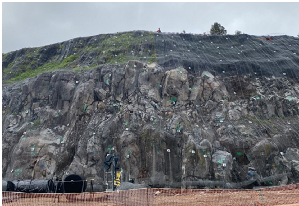
Figure 11.2. Final rock slopes with rock bolts and mesh
