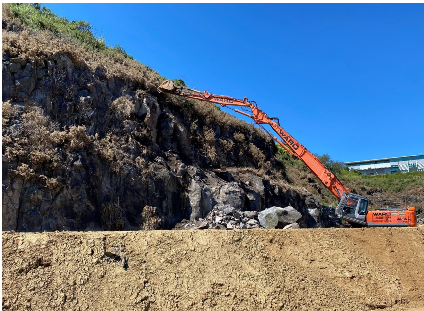
Figure 8.1. Scaling using an excavator to reduce rockfall risk at the Kauriki/Korere Terrace development in Stonefields
