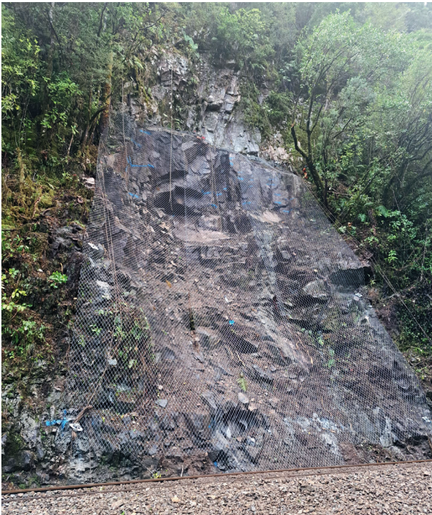
Figure 6.45. A simple drapery mesh system installed adjacent to a railway line (KiwiRail, 2023)
