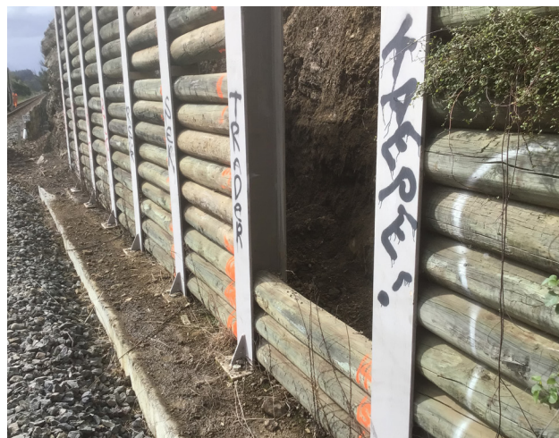
Figure 6.38. An example of the ease of clearance of a TDX Wall
