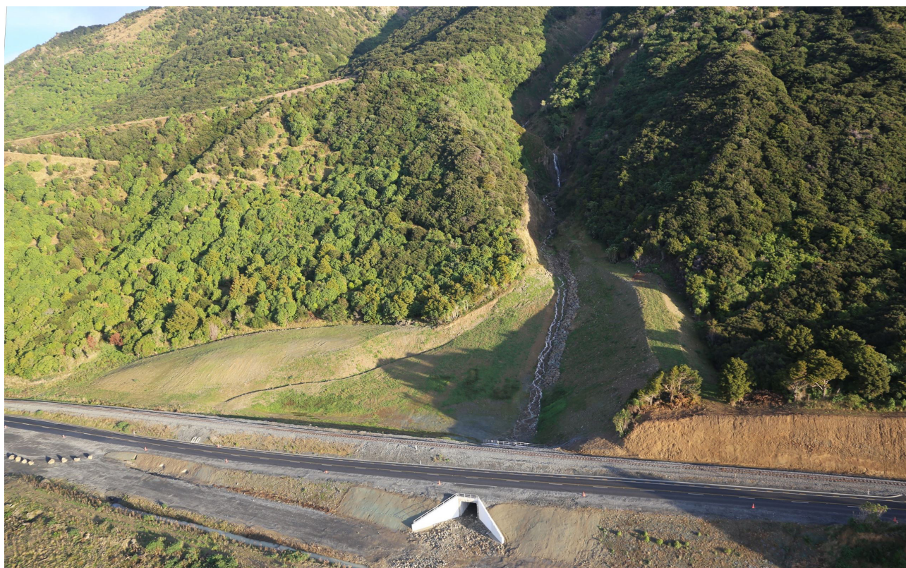
Figure 6.29. An example of a large catch area basin for debris flows and landslides, Kaikōura, New Zealand (NCTIR, 2019)
