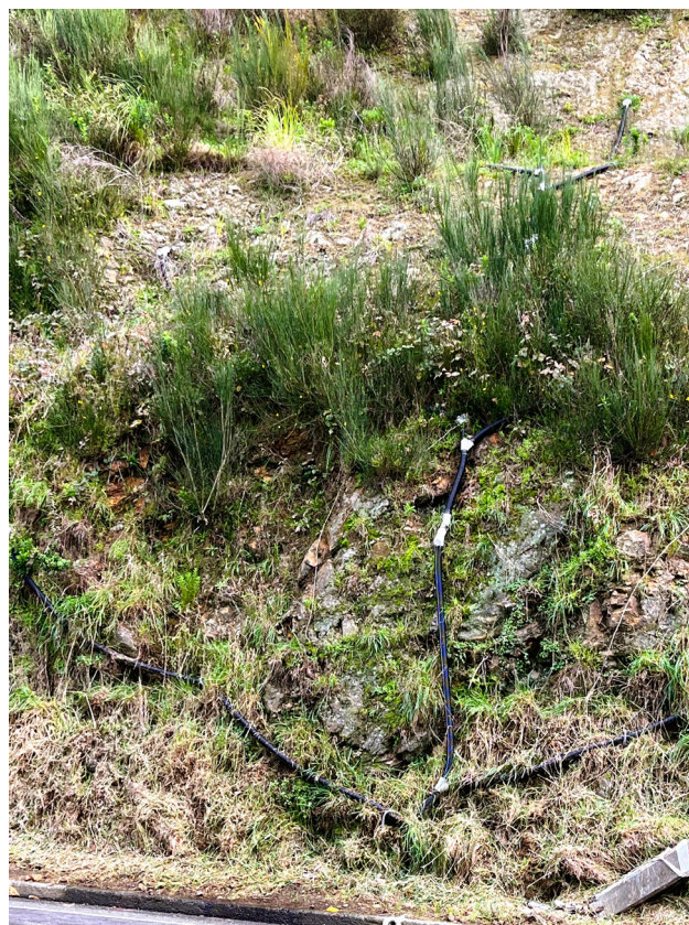
Figure 6.28. A series of horizontal drains connected by surface pipework to a discharge point into the stormwater network on a rock slope in Wellington
