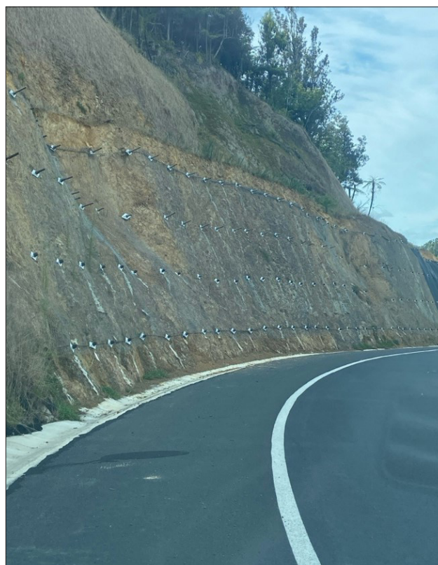
Figure 6.9. Soil nail stabilisation works at Brynderwyn Hills, SH1 Northland
