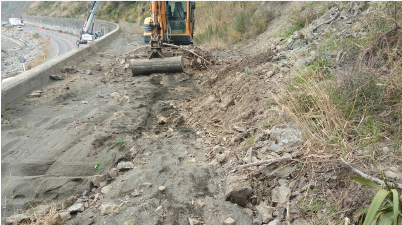
Figure 6.53. An example of the placement of pea-gravel (AP19 or similar) to act as a dampening material above a tunnel/rockfall shed
