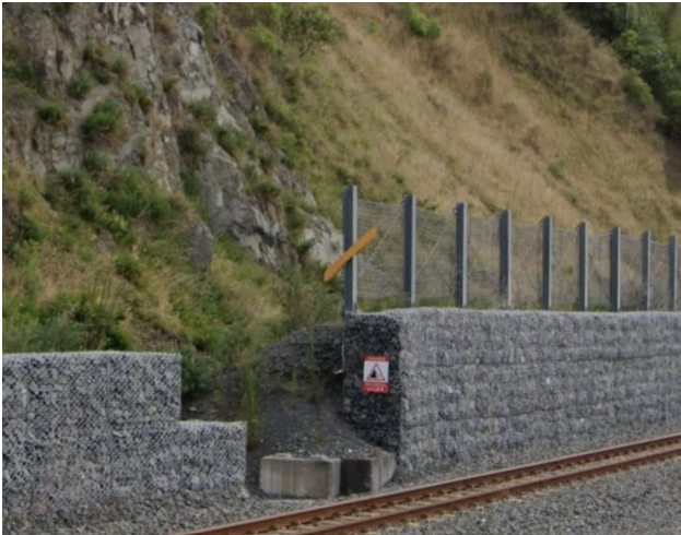
Figure 6.31. An example of a clearance marker used to indicate location and angle of structure, Kaikōura (NCTIR, Google Streetview, 2024)
