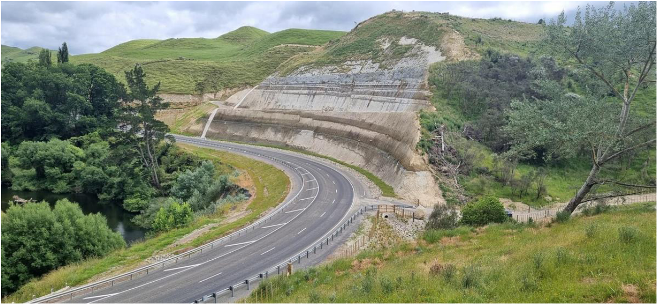
Figure 8.5. SH4 between Whanganui to Raetihi involved retreating into a hill following a 2015 landslide (NZTA, 2023)
