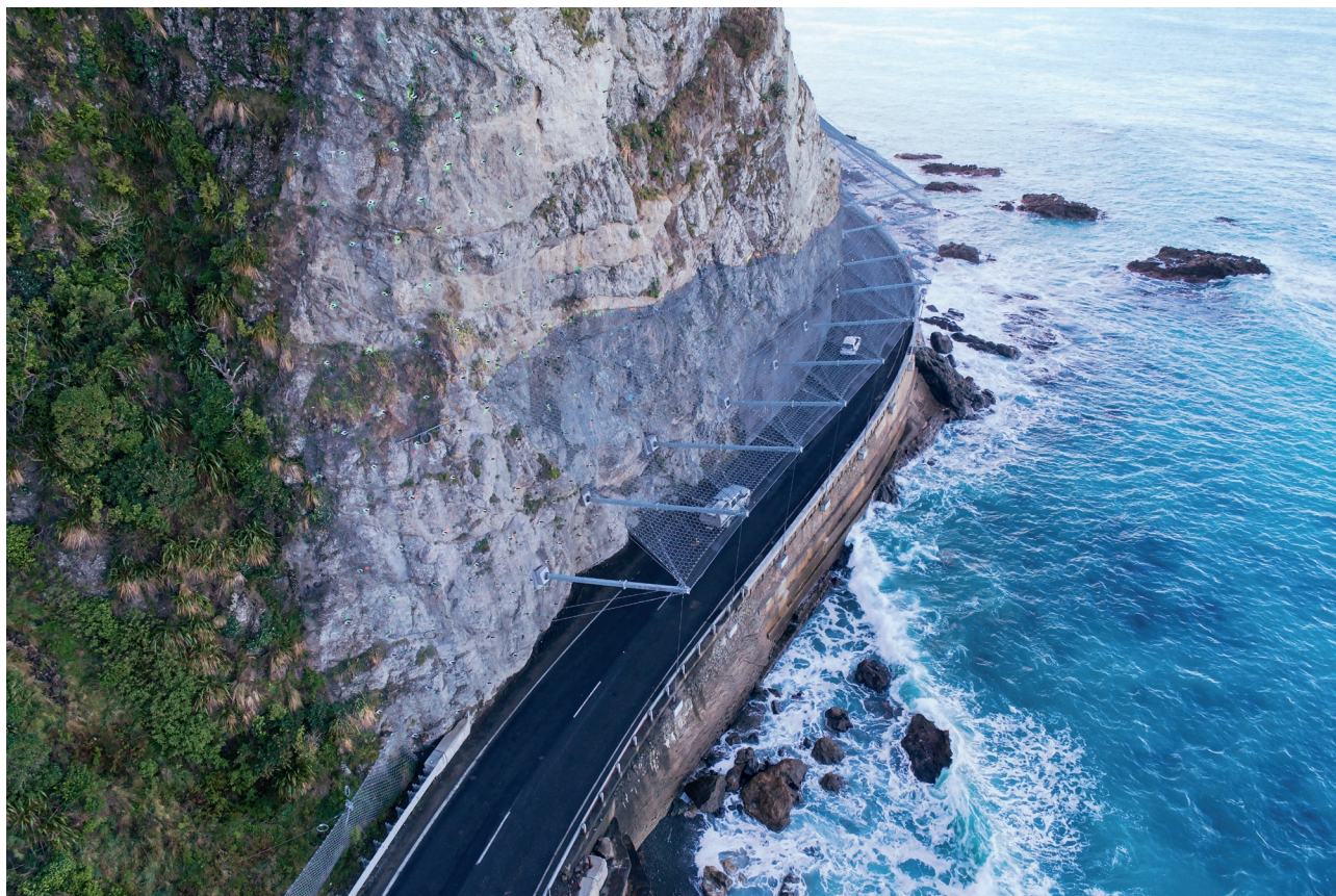
Figure 6.52. An example of a rockfall canopy installed across a State Highway to mitigate the rockfall from a near-vertical sea cliff, Kaikōura (NCTIR, 2021)
