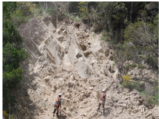
Figure 6.19. Rock scaling works in jointed rock in Maitai Valley, Nelson (Source: Ground Anchor Systems Limited)
