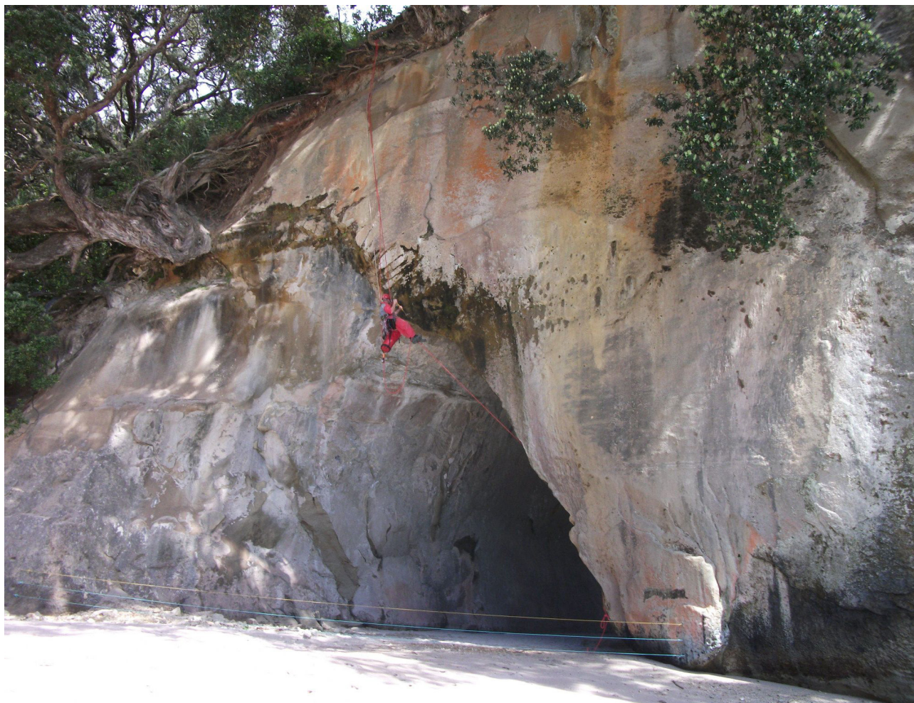
Figure 8.4. Scaling undertaken by rope to remove the rockfall risk at Cathedral Cove
