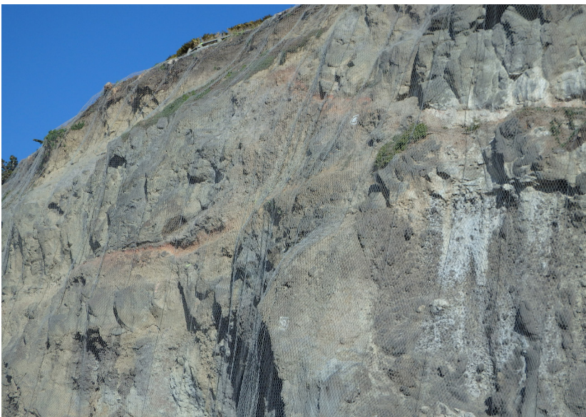
Figure 6.46. A drapery mesh system in Clifton Terrace, Christchurch (Photo courtesy of Eric Ewe)
