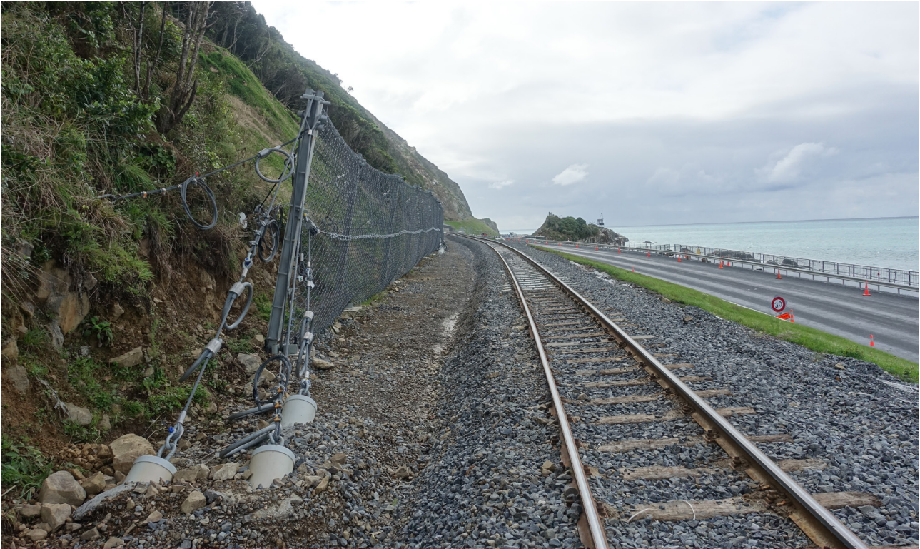
Figure 6.41. An example of the use of a middle transmission rope on an SL-150 Geobruigg Shallow Landslide barrier to reduce deflection into the rail corridor, Kaikōura (KiwiRail, 2023)
