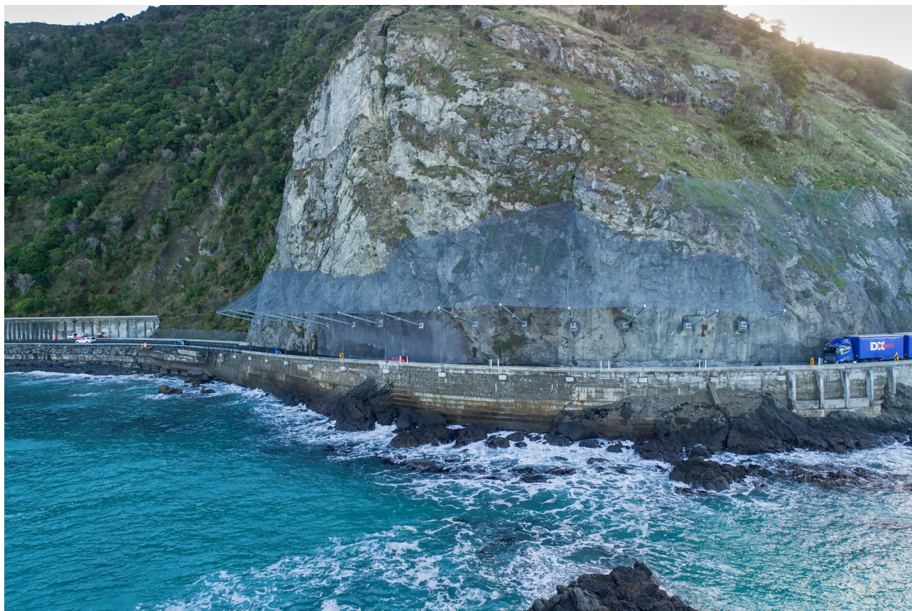
Figure 6.55. An example of the Southern Hemisphere's first dynamic rockfall canopy, Kaikōura (NCTIR, 2021)
