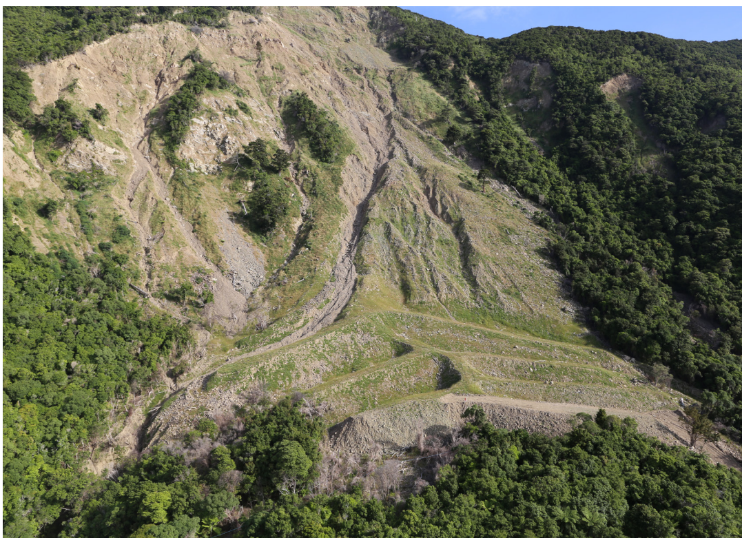
Figure 6.40. An example of on-slope diversion bunds used to redirect debris. These require careful consideration of maintenance to maintain functionality and access for constructability, and ongoing inspections and repairs
