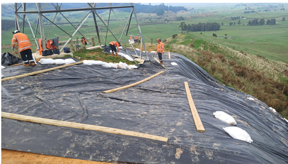
Figure 8.3. Plastic membrane sheeting used to prevent immediate ingress of stormwater into an active slip site in a vicinity of a transmission tower (Source: Northpower, 2024)
