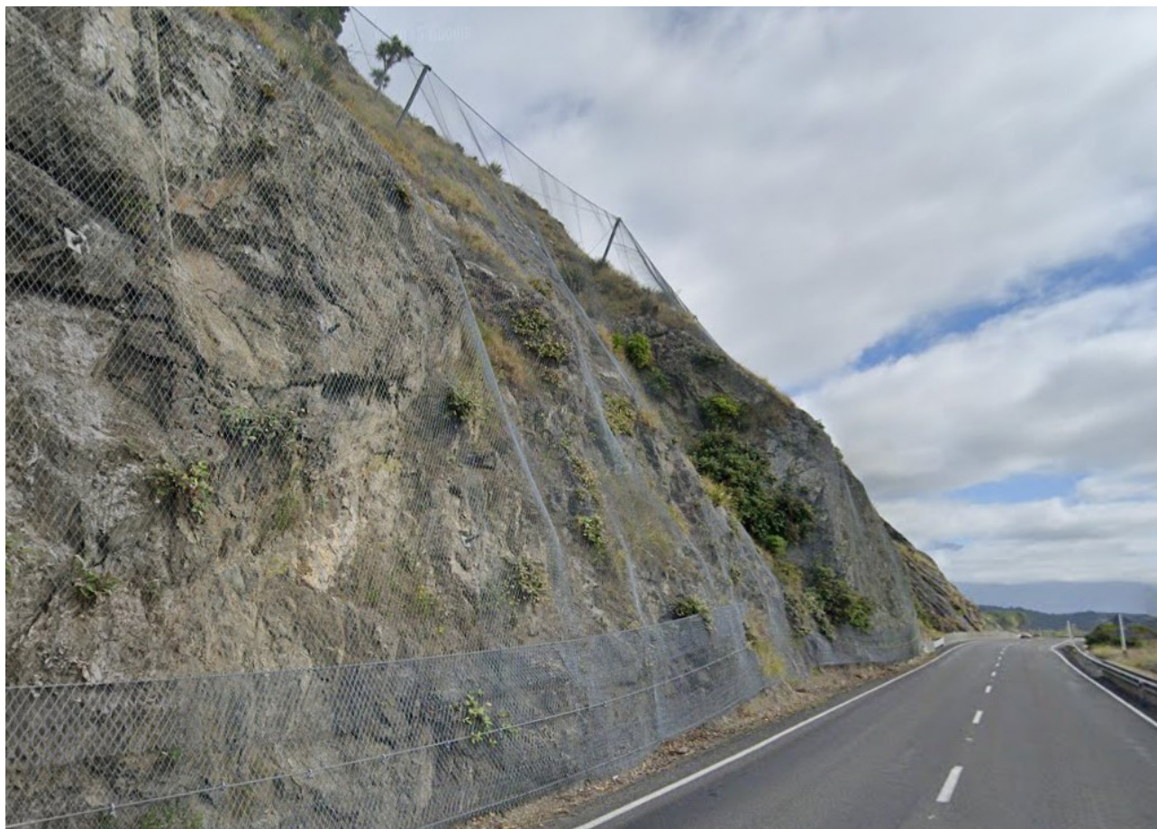
Figure 6.50. An example of an attenuator installed close to the roading corridor, with additional retention cables and mesh at the base to reduce deflection. Kaikōura (Google Streetview, 2024)
