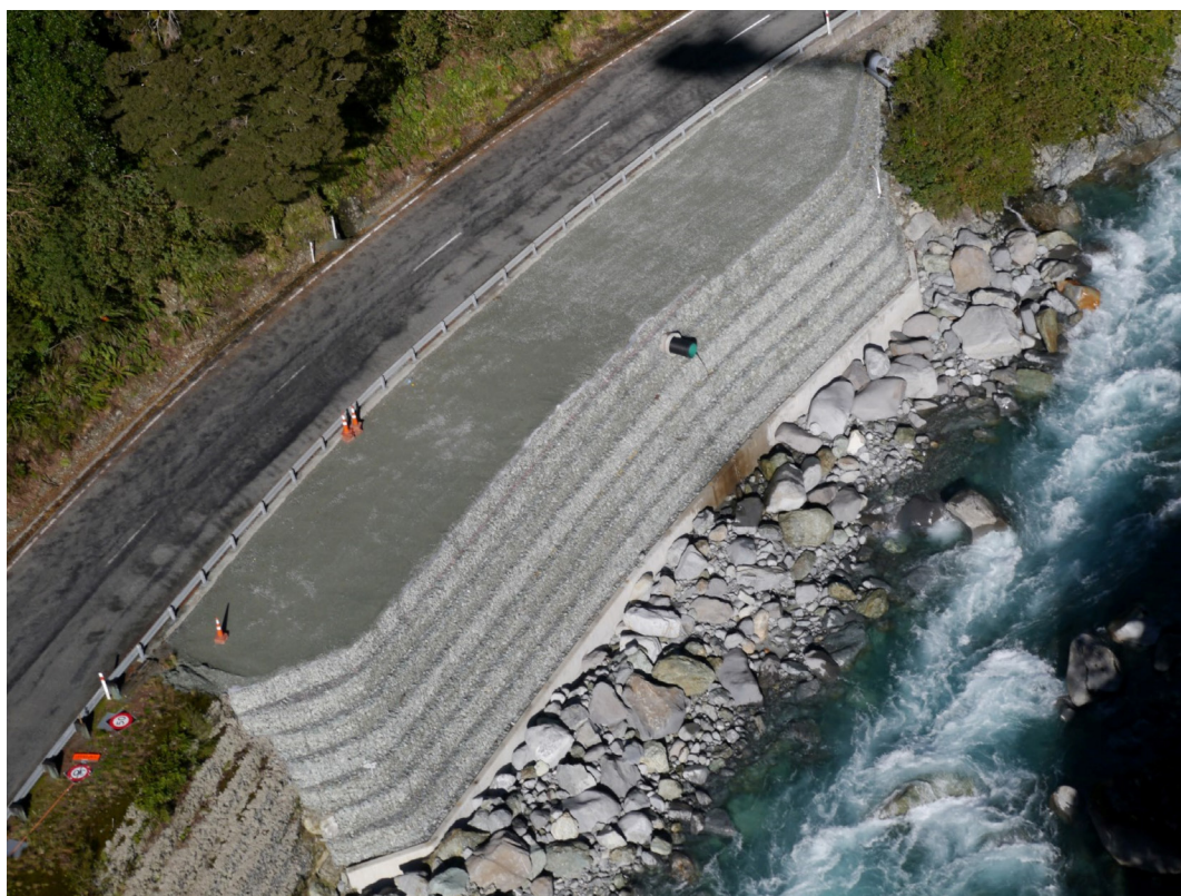
Figure 6.24. Gabion-faced reinforced soil wall buttressing the road and stabilising a landslide on Milford Road, Milford Sound (Photo courtesy of Eric Ewe).
