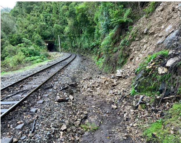
Figure 6.33. A typical rail-side catch ditch to retain minor rockfalls, Stillwater to Ngakawau Line (KiwiRail, 2023)
