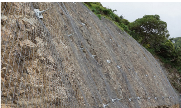
Figure 6.26. High-capacity steel mesh (Tecco) installed over highly fractured greywacke (Source: Geovert Limited)
