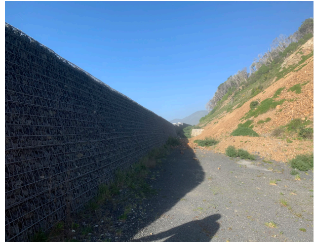
Figure 6.32. A larger catch area integrated with a bund, Kaikōura (NCTIR, 2019)
