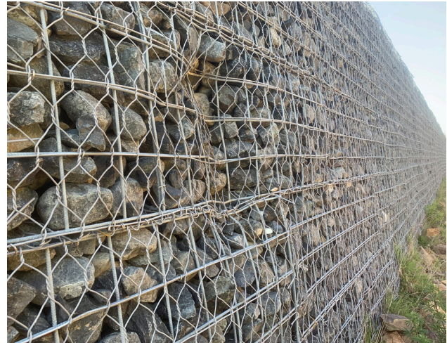
Figure 6.35. An example of a deformable MSE bund, with deformation observed from a recent rockfall impact, Kaikōura (NCTIR, 2020)
