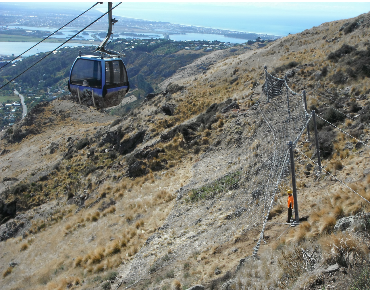
Figure 6.49. Attenuator fence in the Gondola, Christchurch (Photo courtesy of Eric Ewe)
