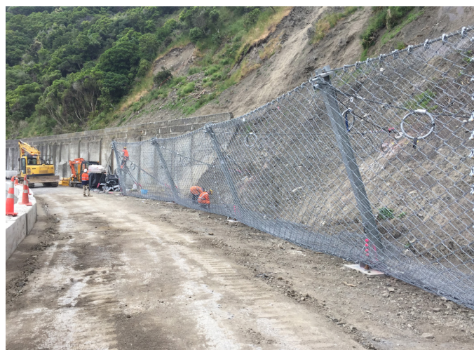
Figure 6.44. An example of a newly completed proprietary (Geobrugg) rockfall and shallow landslide barrier, Kaikōura (NCTIR, 2018)
