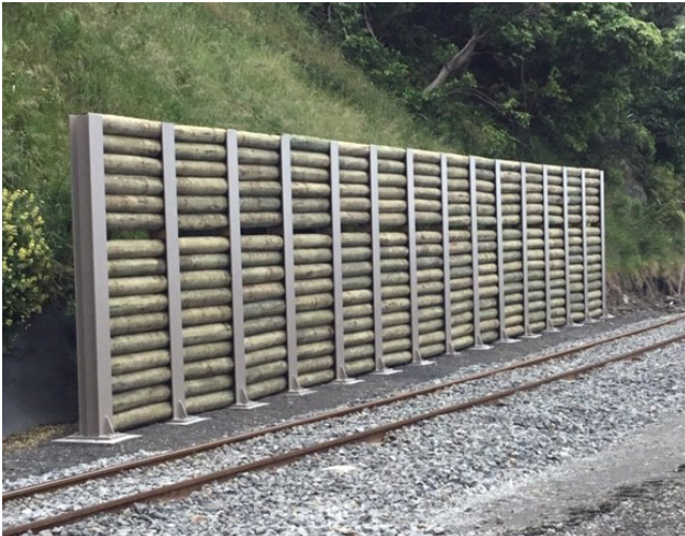
Figure 6.34. An example of a non-deformable, Timber Debris Interception (TDX) Wall, Kaikōura (NCTIR, 2020)
